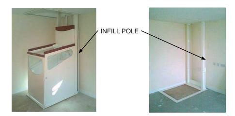
If the gap between the rear of the guides and the wall exceeds 120mm then an infill pole will be required as shown above.
